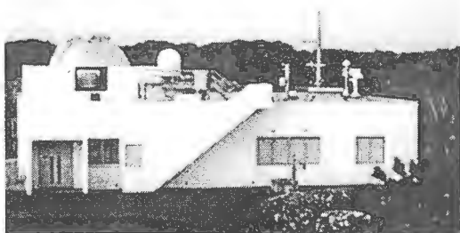
Exterior of GUTS-SLR facility
