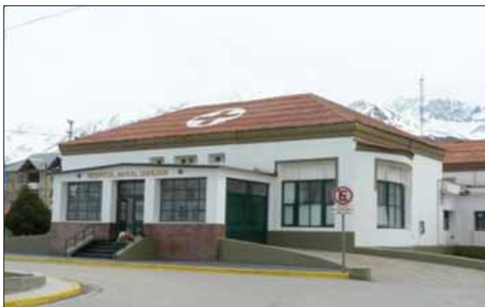
Figura 16. Hospital Regional de Ushuaia.
