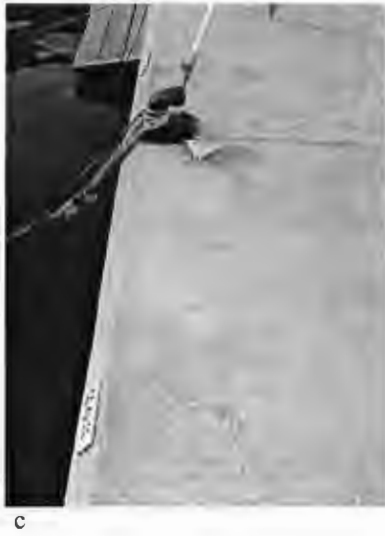
Fig. 17: Control points: bollard n° 15, fire hydrant and bollard between 268 and 269
